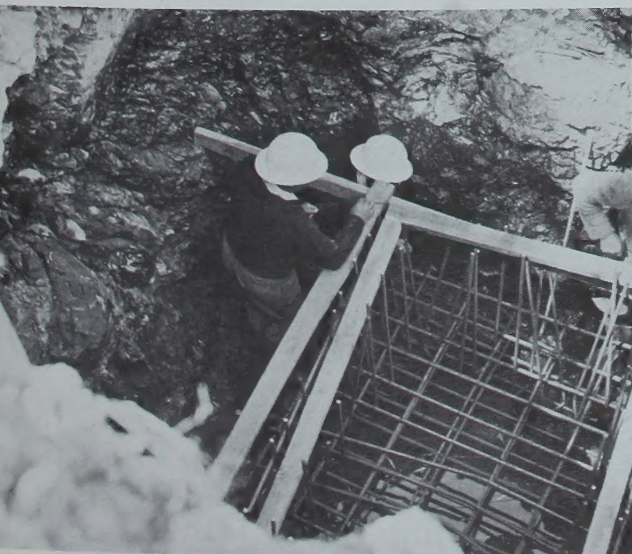
The first reinforcing steel is being placed in position at the bottom of the water supply pump house for the new mill alongside Ironbark Creek.
